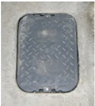
Floor plate cover for backwater valve.
