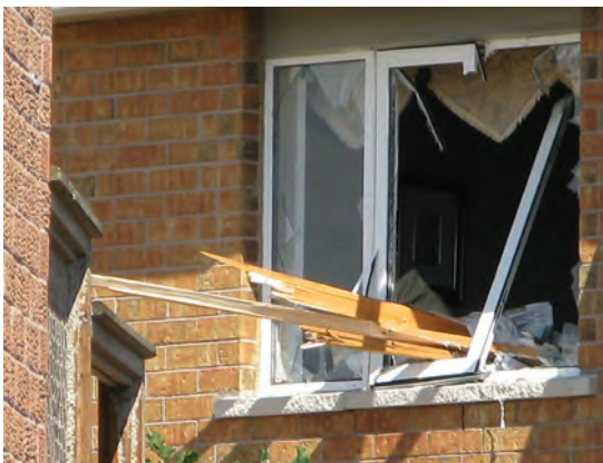
Flying debris from severe winds can easily penetrate unprotected windows.
