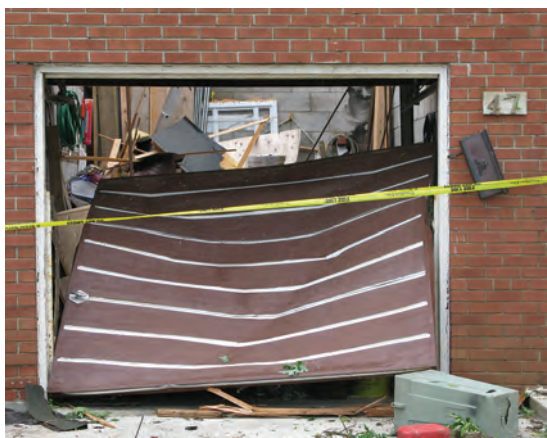
Garage doors can be the weakest opening of a home in a severe wind storm.
