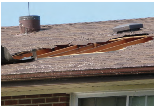
Roof sheathing must be securely fastened to prevent wind damage.
