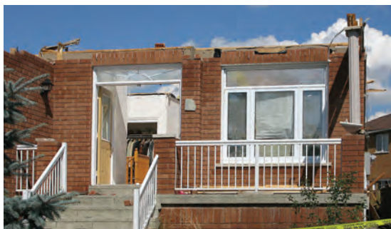
Roof uplift and failure is a common source of damage linked with high winds and tornadoes.
