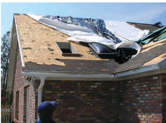
High winds are a major cause of roof damage.
