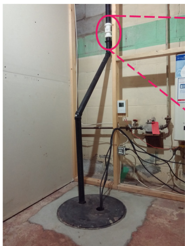
Figure 7: Top: Check valve (Source: Gold Seal Homes) Left: Sump pump system retrofit (Source: Institute for Catastrophic Loss Reduction)
